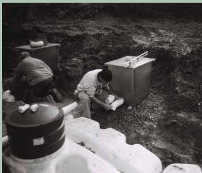
Workers install the rainwater harvesting collection tanks and mixing mechanisms, which are buried underground (top). Installation of the roof washers (bottom). Photos courtesy of Douglas Phillips.
